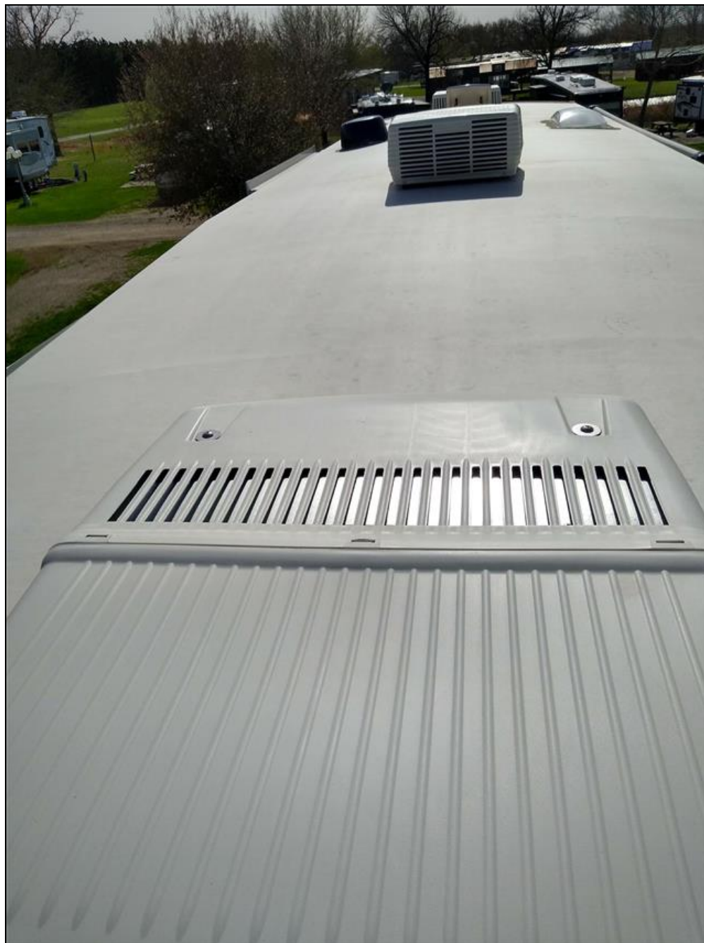
Roof - Back to Front
